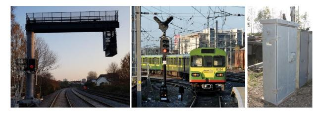
Figure 4-3 Sample DART+ West signalling infrastructure (cantilever, signal, LOC, from left to right)
